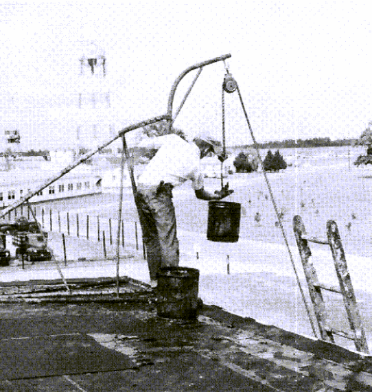
Rehabbing turns old to new
